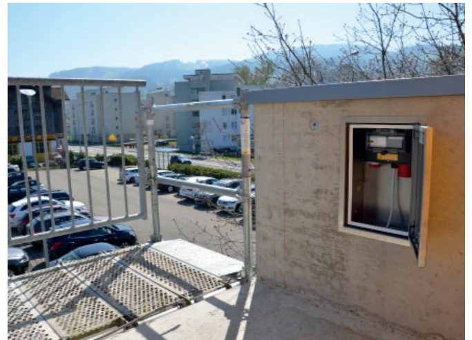
Unobtrusive recessed distribution box
