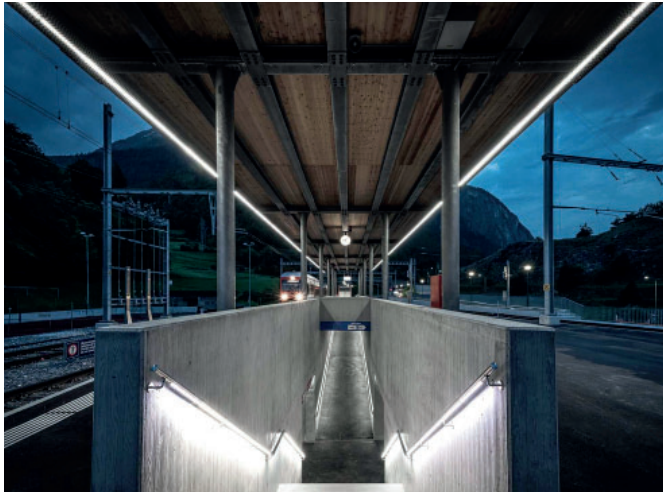
LaneLED WALL and LaneLED INOX42, railway station Sembrancher
