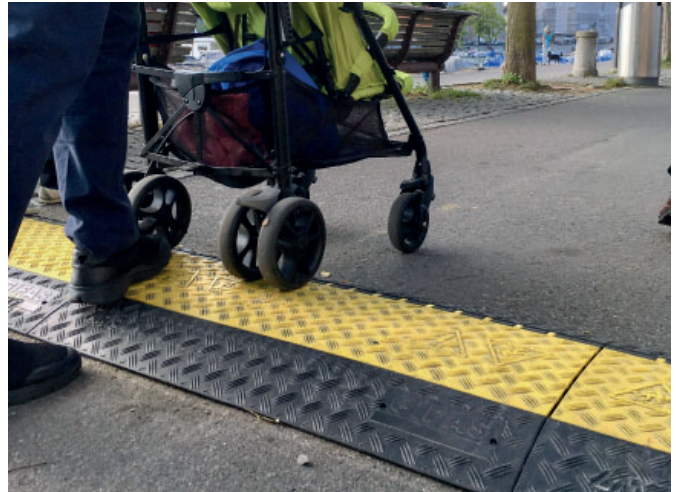
Cable crossover in Zurich
