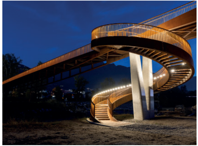
LaneLED WALL, Torretta Bellinzona footbridge
